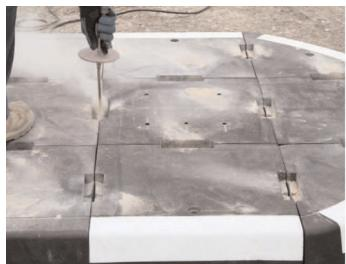
**4.** Blow out anchor holes using a long-nosed air gun, powered by a 120-psi portable compressor. Insert resin starting at base of hole, 2 to 3 pumps required using a resin gun.
