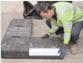
**2.** Mark position on road for location of medians and assemble the Redipave modules accordingly.
