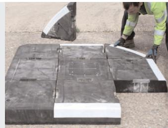
**3.** Ensure all module joints are butted tightly together. Start from the middle sections of the RediPave, and with a 19/32-in. drill bit, drill through the holes to a depth of 10.5 inches or greater. The drill used will be an electric Hilti T15 or T21 hammer drill (or similar) powered by a generator and a suitable power extension cord.
