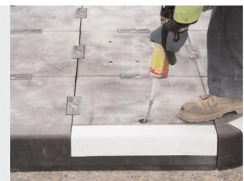
**6.** Repeat drilling, blowing, and resin for remaining middle holes and use black plastic anchor block to secure median. Once middle sections have been completed, drill remaining outside holes and blow out anchor holes using the long-nosed air gun. Thoroughly blow out holes and insert resin starting at base of hole, 2 to 3 pumps required per hole.
