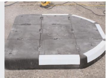
**7.** Insert torx screw and plastic washer into RediPlug. Tap assembly down to 2 3/4-in. above module surface and tighten with impact wrench, ensuring washer is firmly seated.
