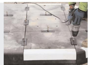
**5.** Insert torx screw through black plastic anchor block and attach RediPlug and tap down to surface level. Tighten with impact wrench; ensuring torx screw is firmly seated.
