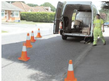
**1.** Insure proper maintenance of traffic is set up to ensure the safety of the workers, motorists and pedestrians.
