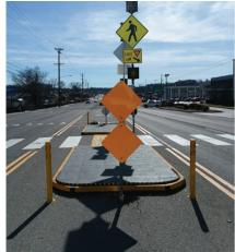
No damage was made to the Modular Medians, even after an automobile ran through 3 sign assemblies.
