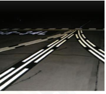
is crucial to the safety of the airfield. Night-time color is evaluated using ASTM D6628.
